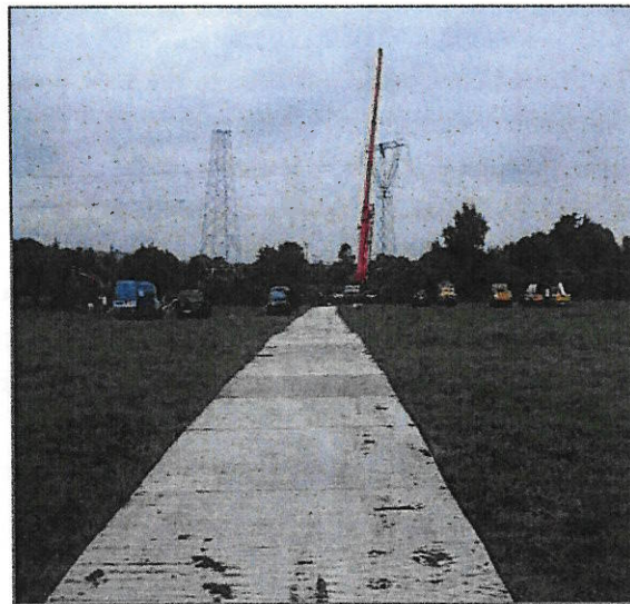
Figure 9 - Temporary Aluminium Panel Tracks
